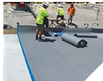
Pre applied (fully bonded)
